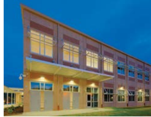
Eastern Guilford features inset brick on its exterior with some additional accents, along with large windows that take advantage of daylighting to save energy costs. Photos: SfL+a.
