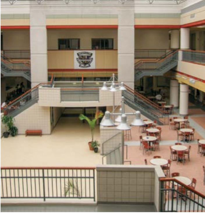
The two-story, 270,568-ft 2 school features a large central atrium that serves as a gathering point for student activities. Photos: Tindall Corp.
