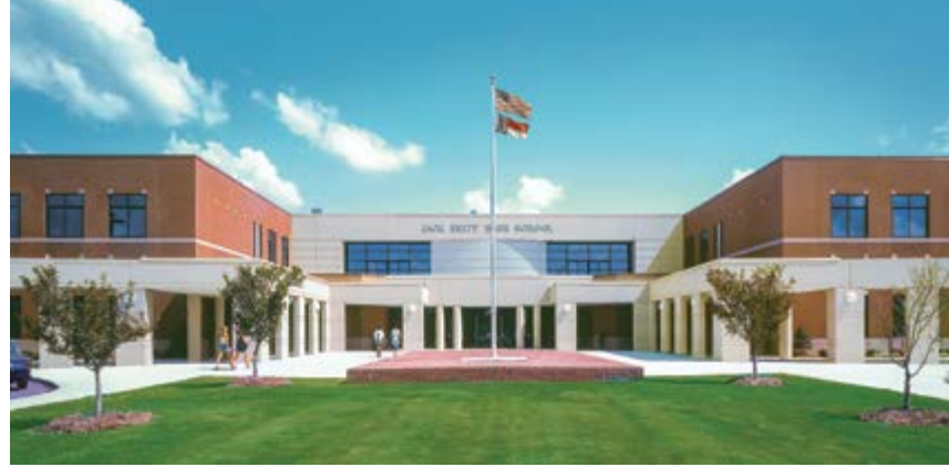
SfL+a’s 1996 design for the Jack Britt High School in Fayetteville, N.C., represented one of the first in the region to use inset thin brick in insulated precast concrete panels. The design garnered positive attention and made precast concrete a strong choice for school façades in the area. Photos: SfL+a.
