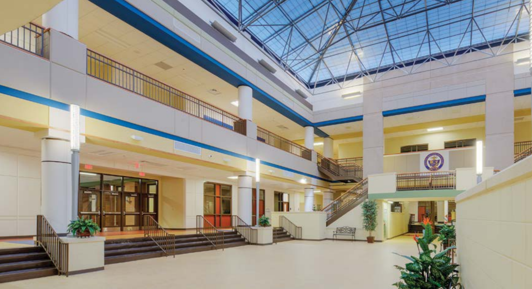
The total-precaster concrete framing system allows long expanses and strong structural support for the atrium, which reflects the design used on the earlier Northern Guilford school. Photos: SFL+a.
