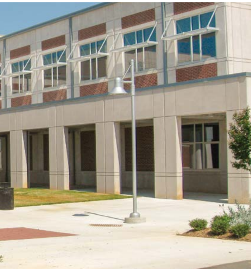
An aggressive schedule and a shortage of masonry labor led designers of the 1600-student Northern Guilford High School to specify insulated, load-bearing precast concrete panels faced with inset brick to clad the building. The panels also provided a hedge against volatile steel prices and provided a low-maintenance panelized system. Photo: Tindall Corp.
